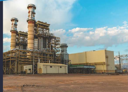
TABAN, 484 MW C. C. Power Plant
