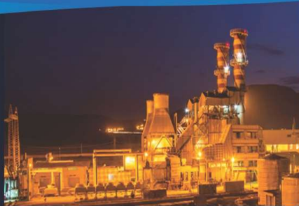
KHOY, 350 MW C. C. Power Plant
